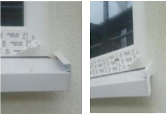
The previous guide may not be added to the existing window frame. Further, the guide may be free of a flow control channel and thus the rainwater may flow along and on the wall face to cause a pollution.
